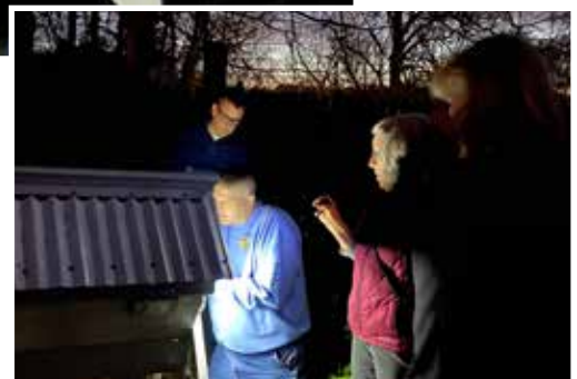
Below: Final steps to installation.
